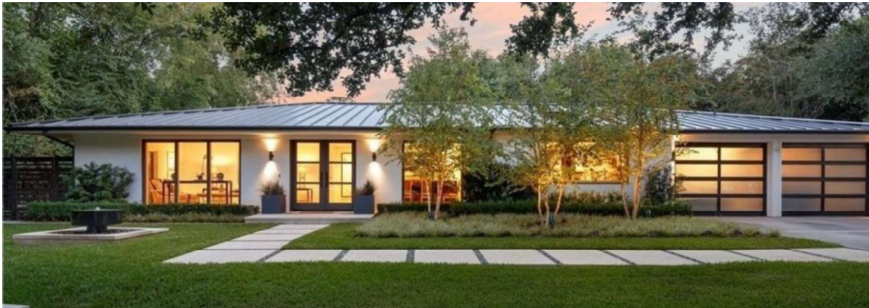
Figure 7 – Modern style house with a low-pitched standing seam metal roof.
