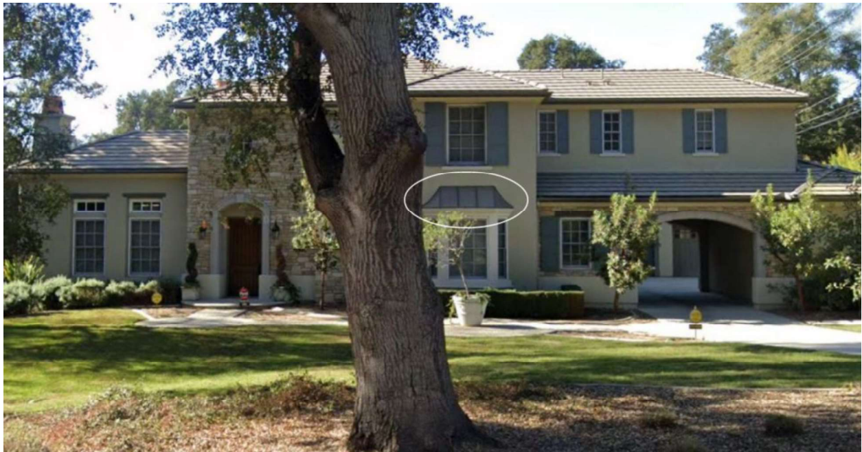
Figure 4 – a French-Country style house with a bay window roof detail consisting of standing seam metal in a dark bronze color.
