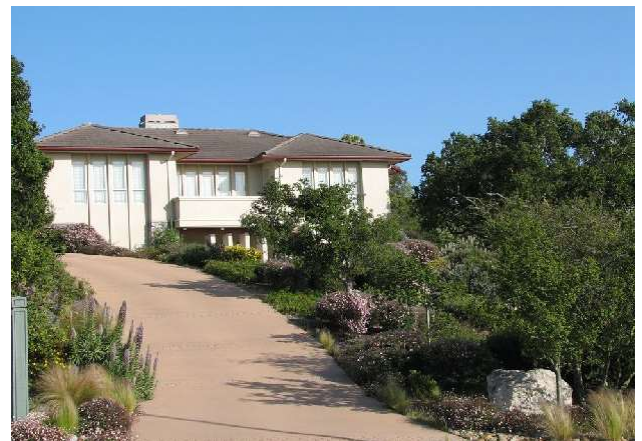
Structure sited to transition with hillside
