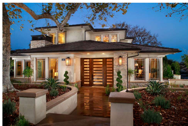
Windows and doors complementary of architectural style
