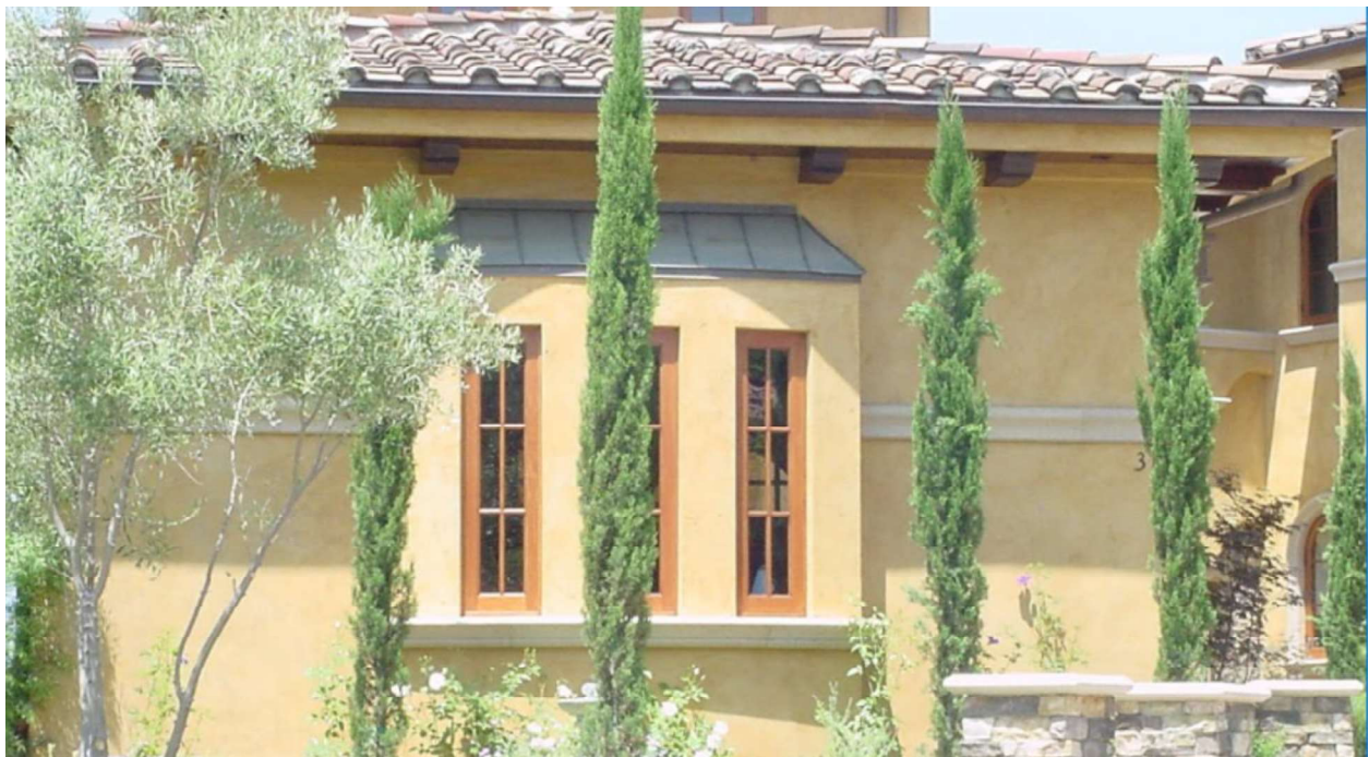
Figure 5 – a Mediterranean-style house with a bay window roof detail consisting of standing seam metal in a dark bronze color.
