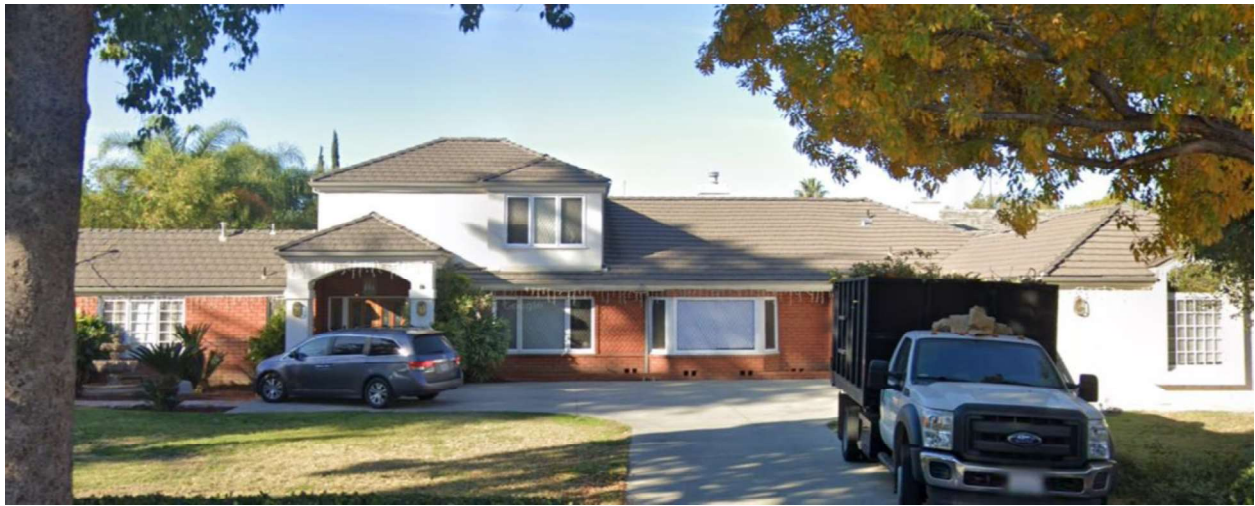
Figure 2 – House at 1231 S. 4th Ave., with existing tile roof.
